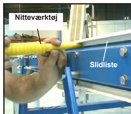
Figur 17: Monter nitten for at fastgøre slidlisten
